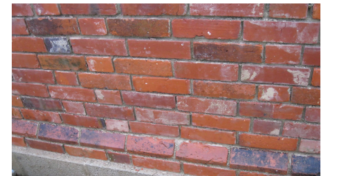
Imperial Swanage Berry Restoration Red Stock brick proposed for walls to match existing brick garden wall
